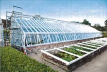
This glasshouse was closed in the summer of 2015 when work started to completely restore it. The glasshouse was cleared, the scaffolding erected and the damaged glass and timbers were removed. Over 130 panes of glass were hand-cut and rotting timbers replaced and painted.
